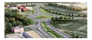
The final element of the Botley Bypass scheme will create a new single-carriageway road running eastwards from Winchester Street, a new bridge crossing the River Hamble and a new roundabout at the A334 junction with the A3051. New and improved pedestrian and cycle routes will also be provided as part of the project, encouraging people to travel more actively, by walking and cycling for their local journeys.
