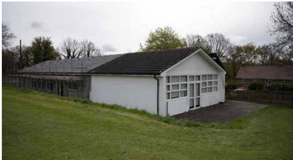
West Meon Village Hall scaffolding photo: A Annabel
